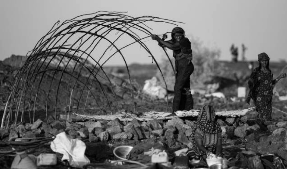
Erecting a hut — called an “arri” — on the lava fields at Saha. Thin branches are bent and lashed together, then covered with reed mats.
